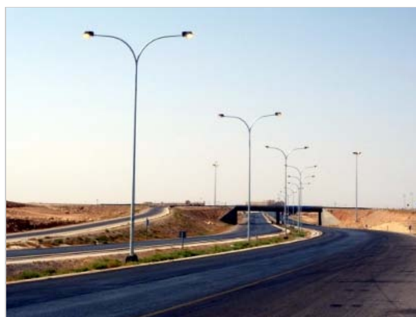
[Figure 4: On the highway south of Amman, Jordan. The lamps are lit, even during the day. Image by Eric Verdeil.]
